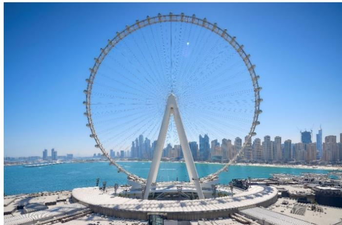
two hubs alone is 40m long, 20m high and weighs over 1,800 tonnes. 11,200 tonnes of steel were used in its construction – one-third more than the quantity used to build the Eiffel Tower. Ain Dubai has 48 cabins for which have the capacity to host 1,750 visitors simultaneously.
